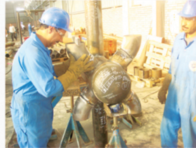
» Piping for El shabab power station project (client Ansaldo).
